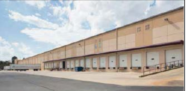
TOTAL - SIX BUILDINGS / 1.6M SF
